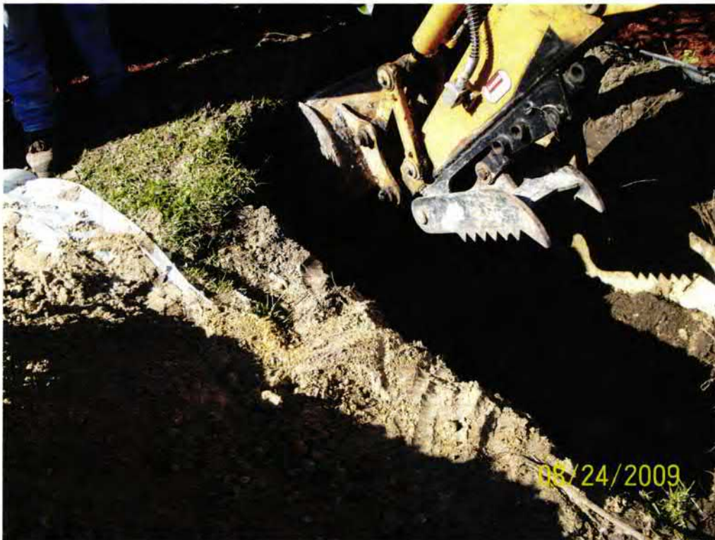
Picture 2: UST 1214Cardinal removal in progress.
